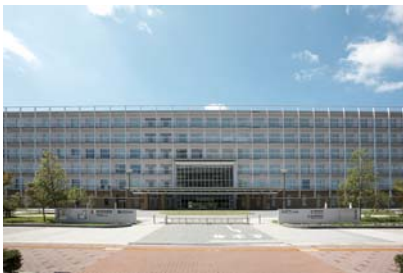
Front of Building
