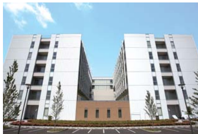
East Side of Building
